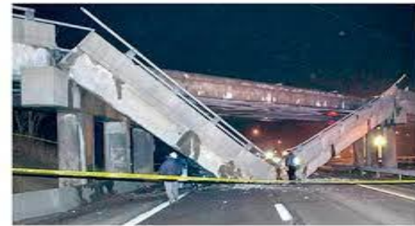
Collapsed Bridge 'Hinge'
