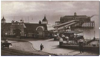
Piers were built to get on and off the paddle steamer.
