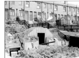
Air Raid shelter
